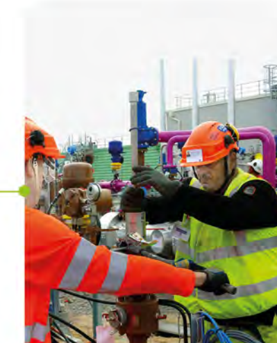
Sampling probe installation
